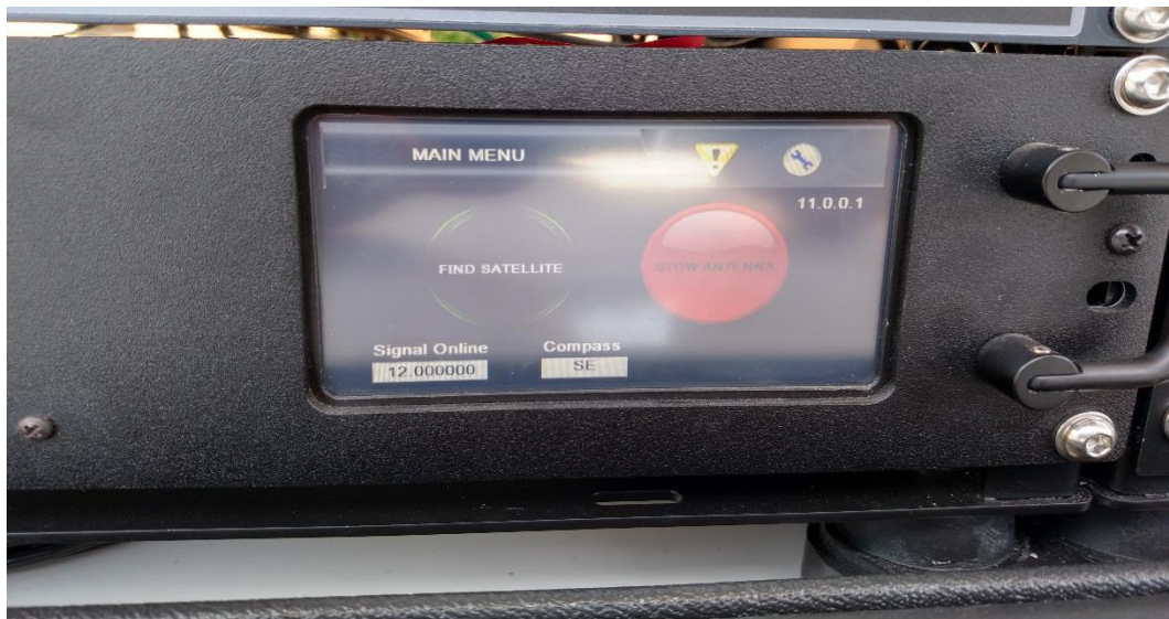
Figure 2 Completed and Connected Screen
